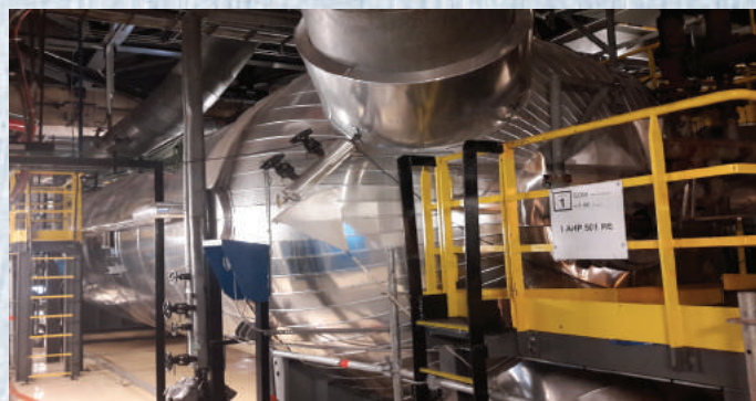
Requalification of AHP heaters at Cattenom NPP (EDF)
