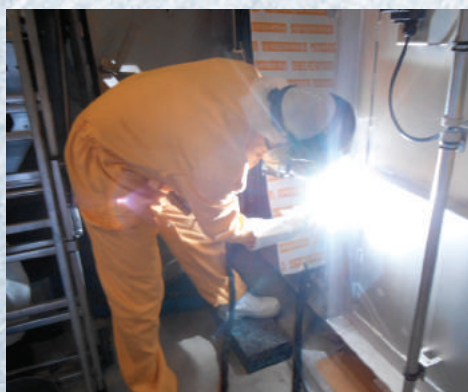
Welding in controlled area of iodine air filter at Paluel NPP (EDF)
