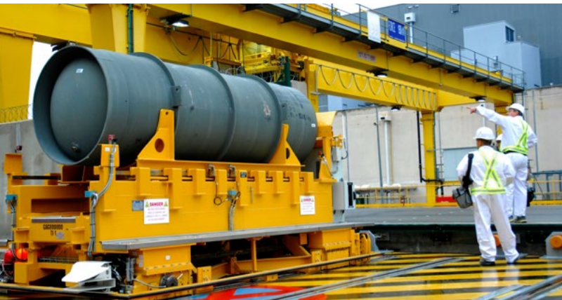
Enriched uranium handling system (GBII plant)
