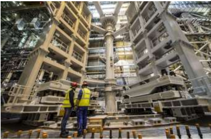
Figure 2: Assembling SSAT No.2 © ITER Org
