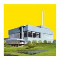
its architecture, which will take the form of a cube without the soaring curves of a typical facility. To fit this design, the flue gas treatment will be placed alongside the boilers instead of further down the line. Meanwhile, the air-cooled condensers will be situated above the machine hall within the main building, rather than on the outside as is usually the case.
