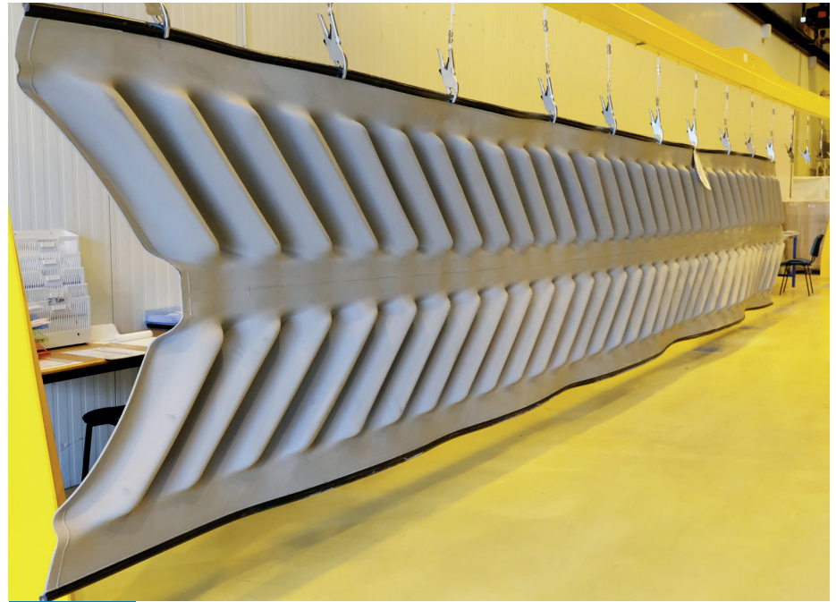
Part of the membrane sealing Chernobyl Safe Confinement.
